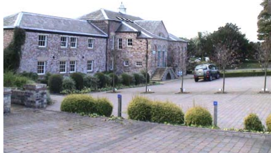
Hesselwood Business Park Hull
